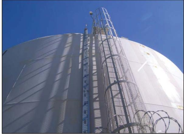
As part of our survey, HDR will determine proper polarization of the internal surface of the reservoir by allowing it to depolarize for a minimum of 10 minutes. This will allow a baseline, native potential, which will be used to determine if the reservoirs are cathodically protected.
