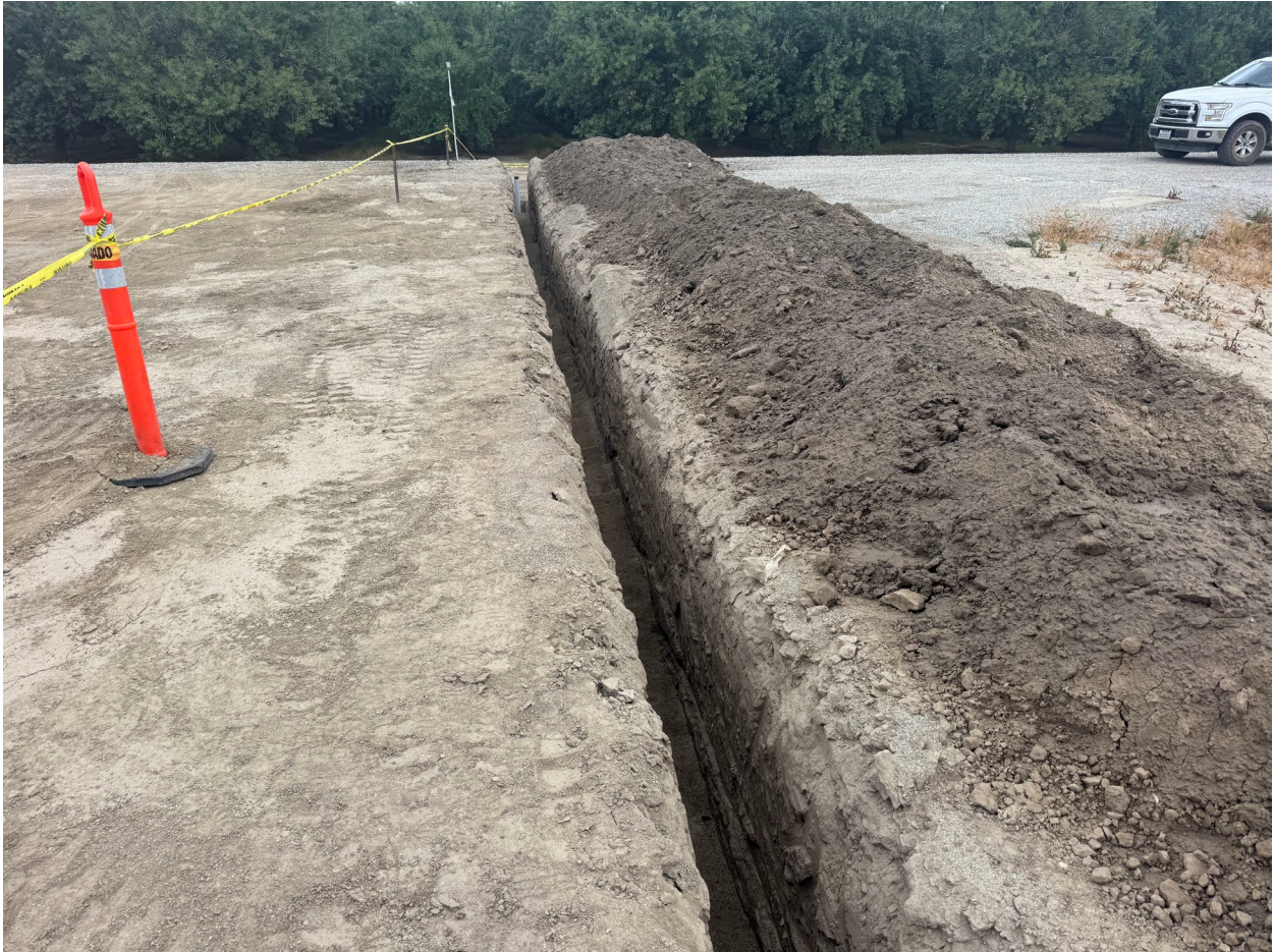
Conduit Installation for Electrical Service at SN-1
