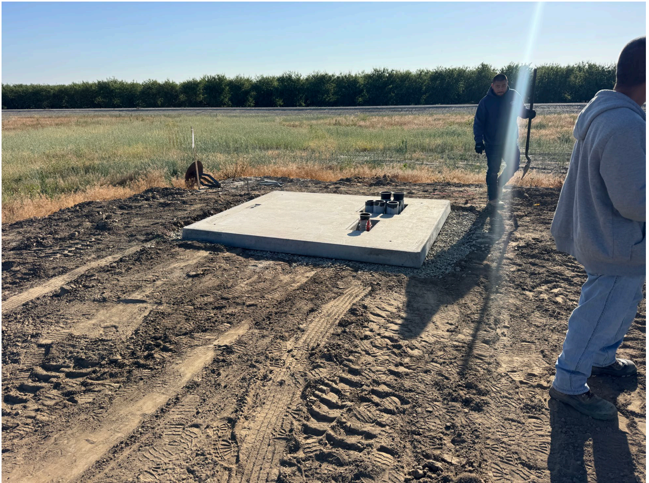
Installing Transformer Pad for SN-2
