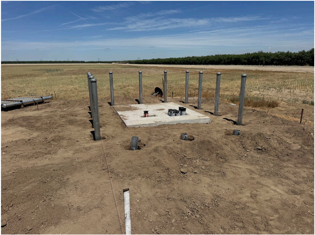
Bollard Installation at SN-2
