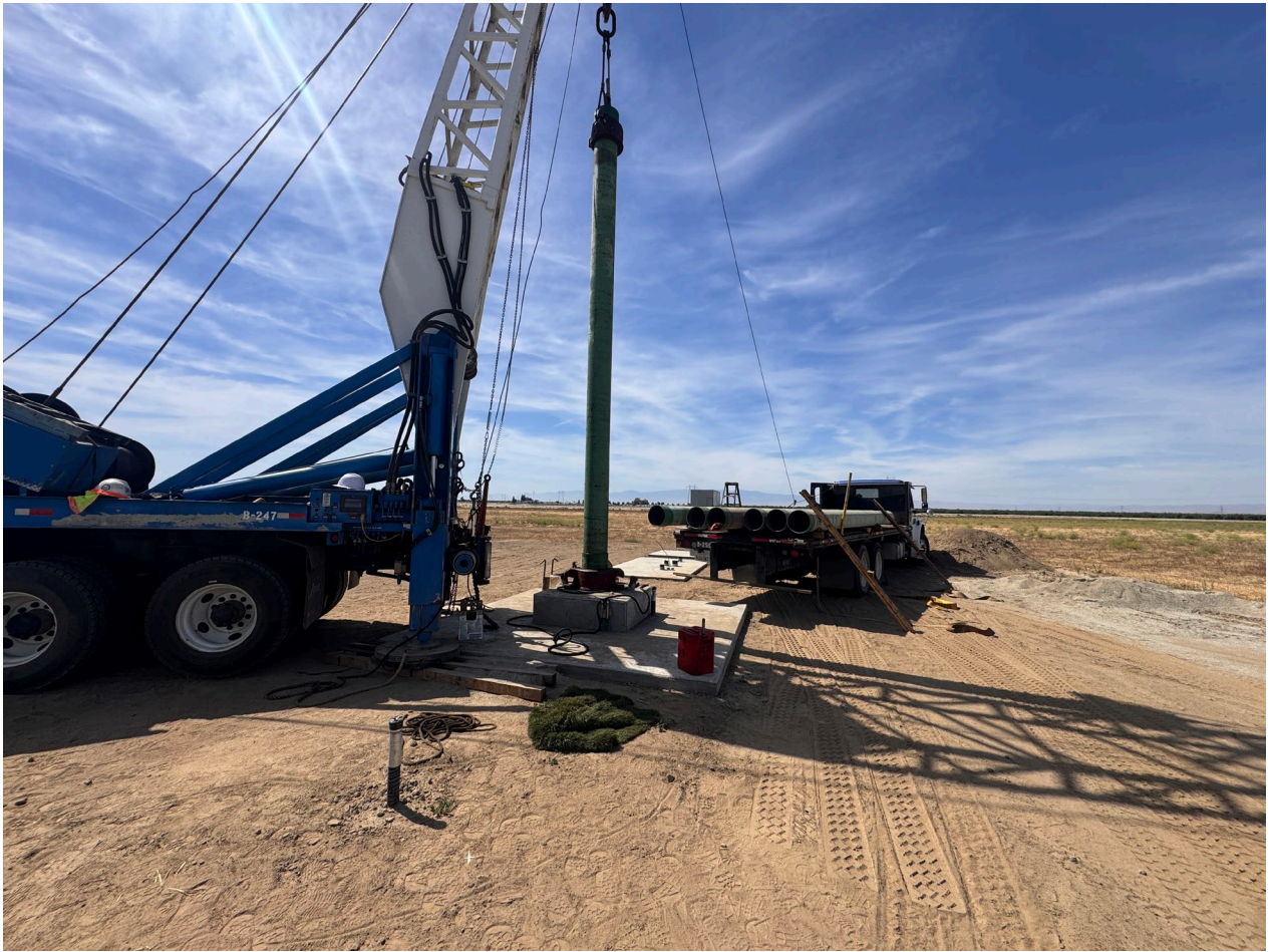
Installing Pump at WE-1
