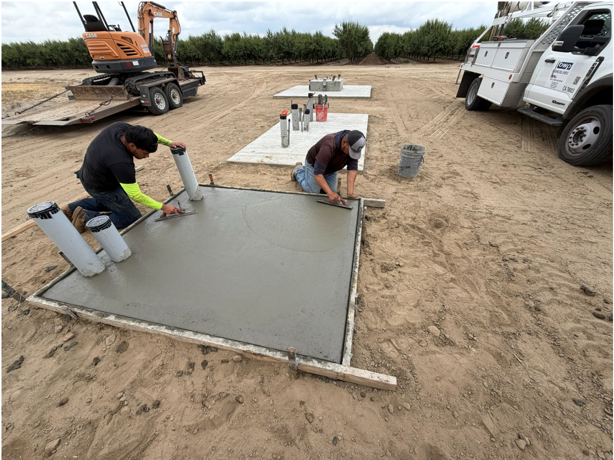
Pouring Meter Pad at WE-1
