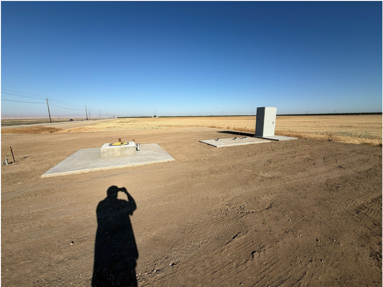
Meter Panel Installed SN-2 (and Installed at All Sites)
