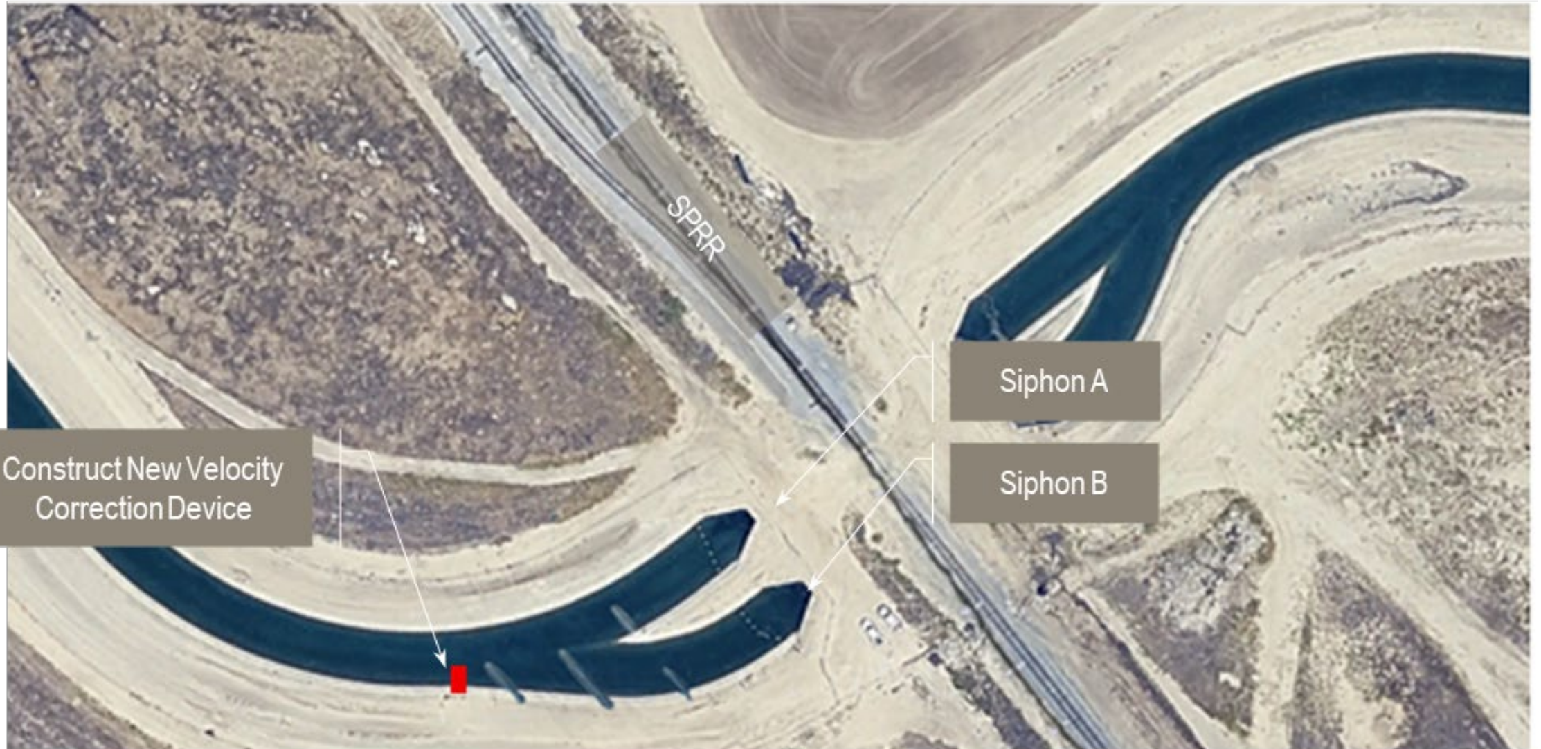
CVC Pool 3 SPRR Siphon Improvements
