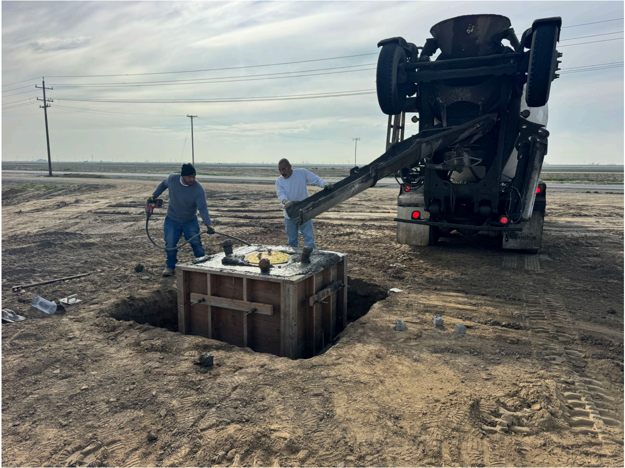
Placement of Well Foundation for SN-2
