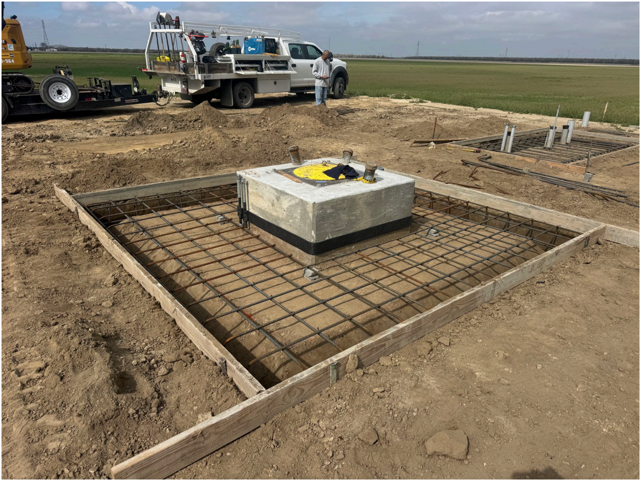
Placement of Reinforcement Steel at SN-2
