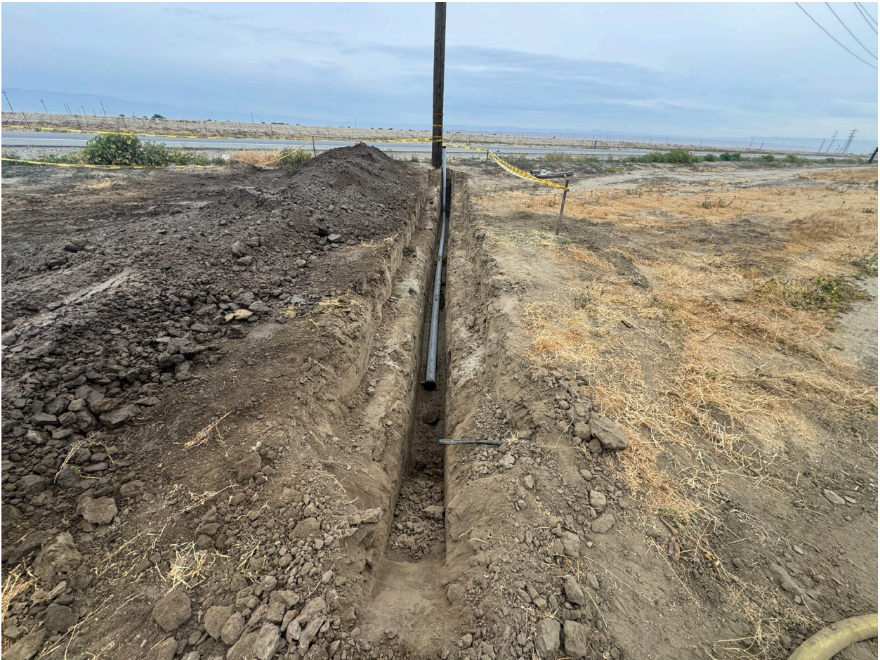
Conduit Installation for Electrical Service at SN-2
