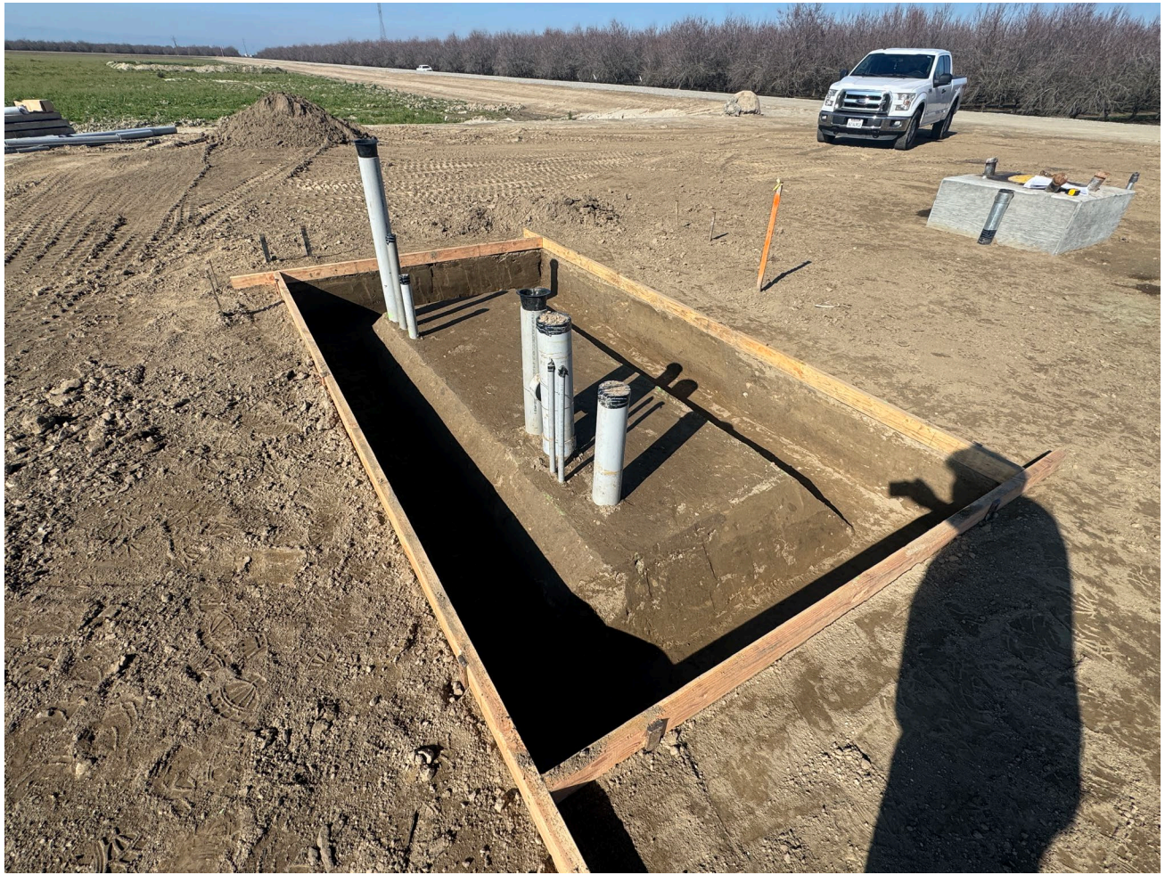
MCC Pad and Well Foundation at SN-2
