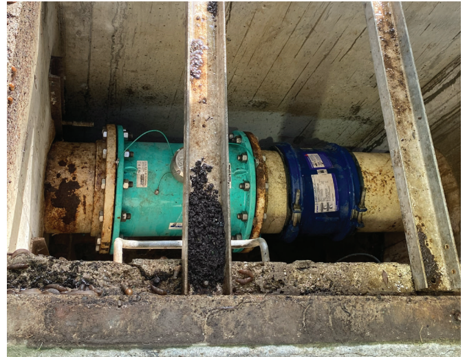
View of Flow Meter Vault with 12-inch flow meter assembly.
