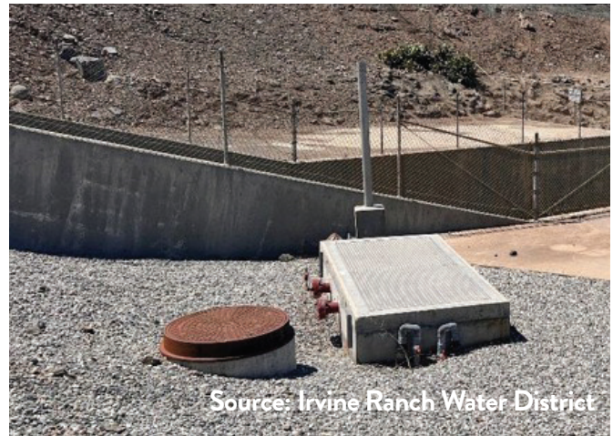
View of Valve Vault structure located just downstream of Villa Park Dam.
