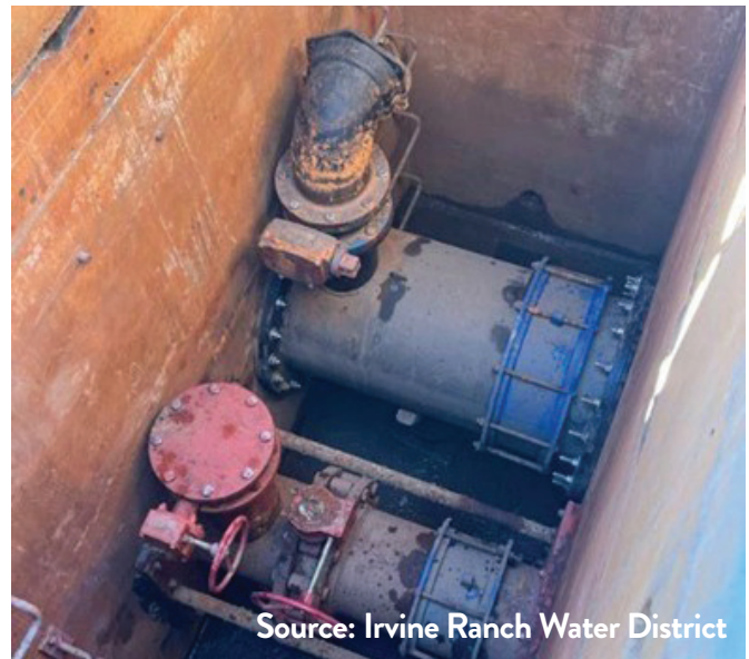
View of piping and valve configuration within the Valve Vault.
