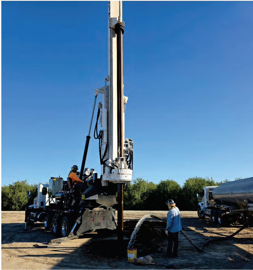
Conductor Casing Drilling
