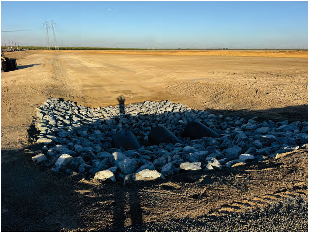
West Enos Crossing Outlet Rip-Rap
