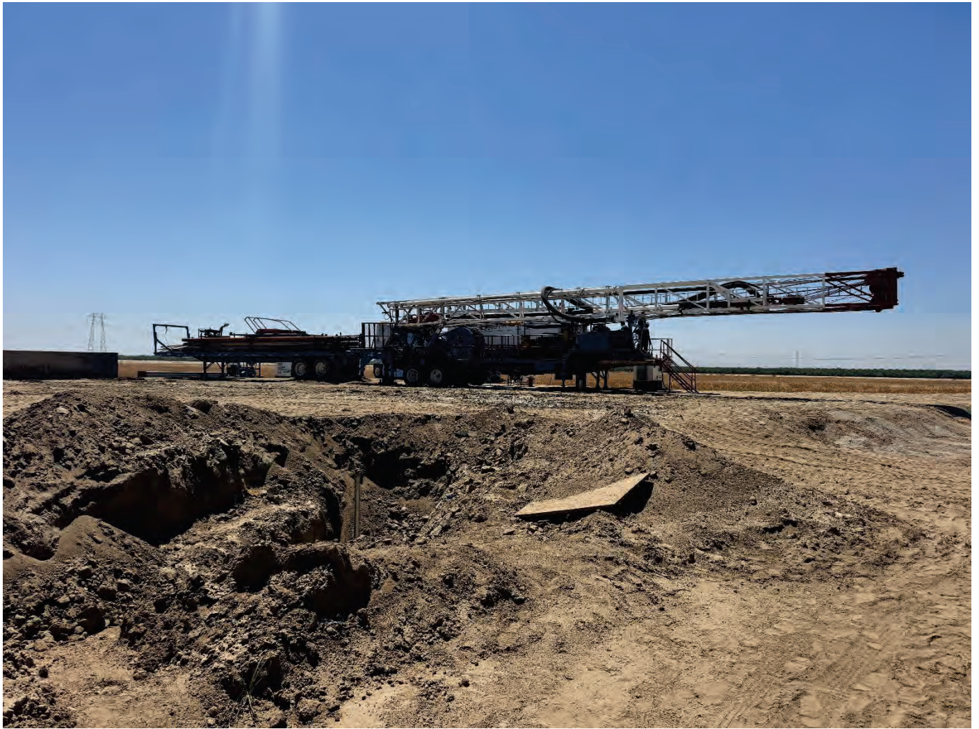
Removing Rig from the Site
