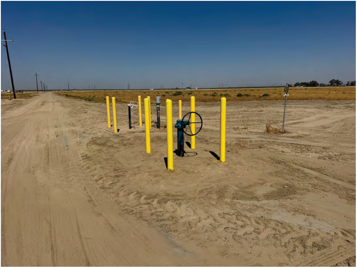
Bollard Installation
