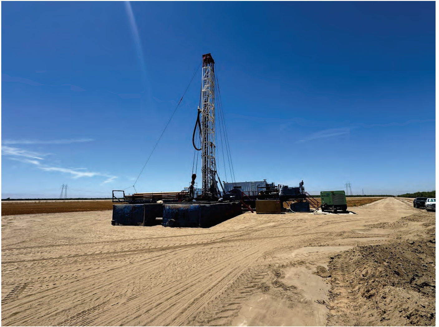
BW&P Mobilizing to West Enos Well #1 Site
