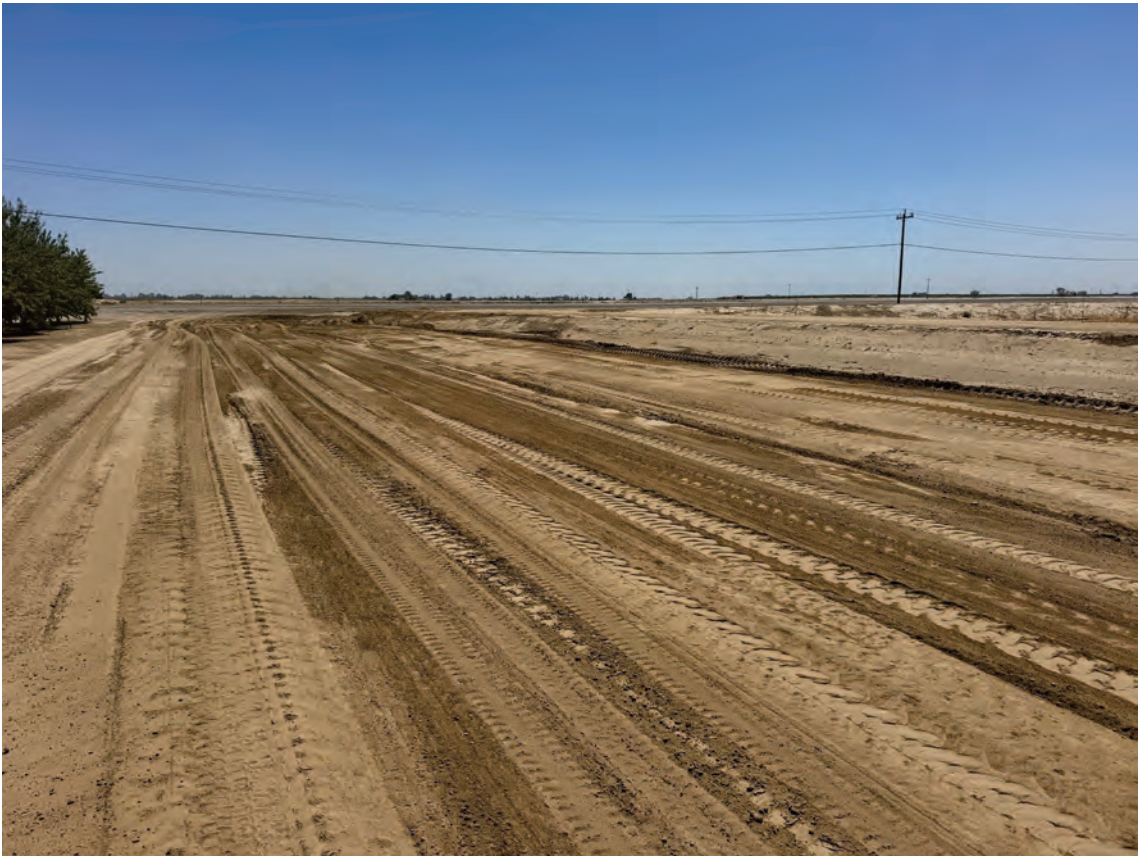
Fine Grading of Pipeline Alignment
