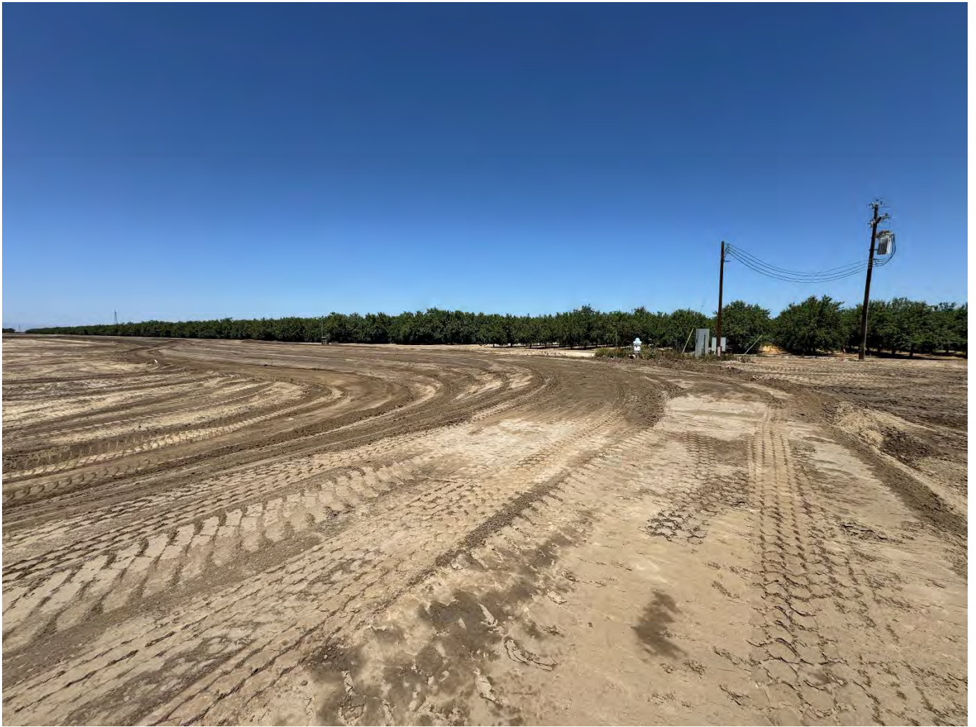
Embankment Built to Final Elevation at Northeast Corner of Property
