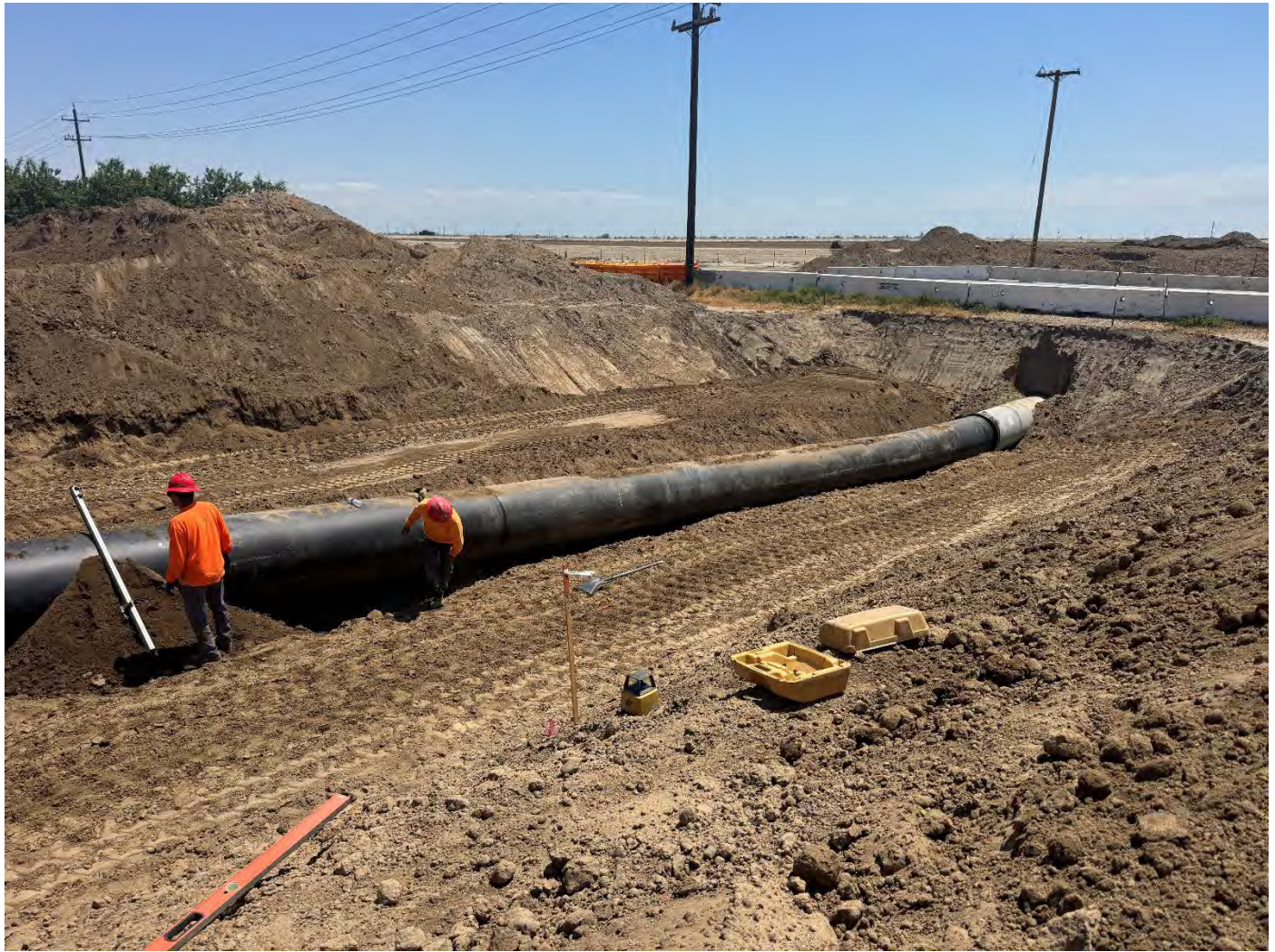
Backfilled Bore Pit, Preparing Pipe for Slurry Backfill
