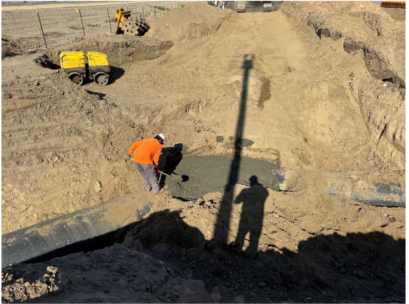
Installing Thrust Block for 45-Deg Fitting
