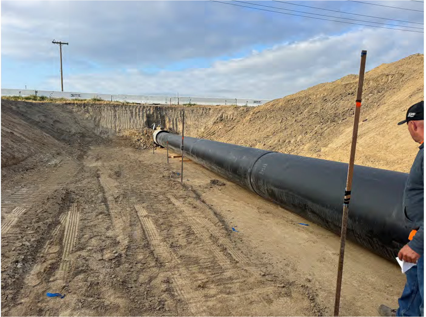
Layout for Backfill of Bore Pit and Pipe Marked Out
