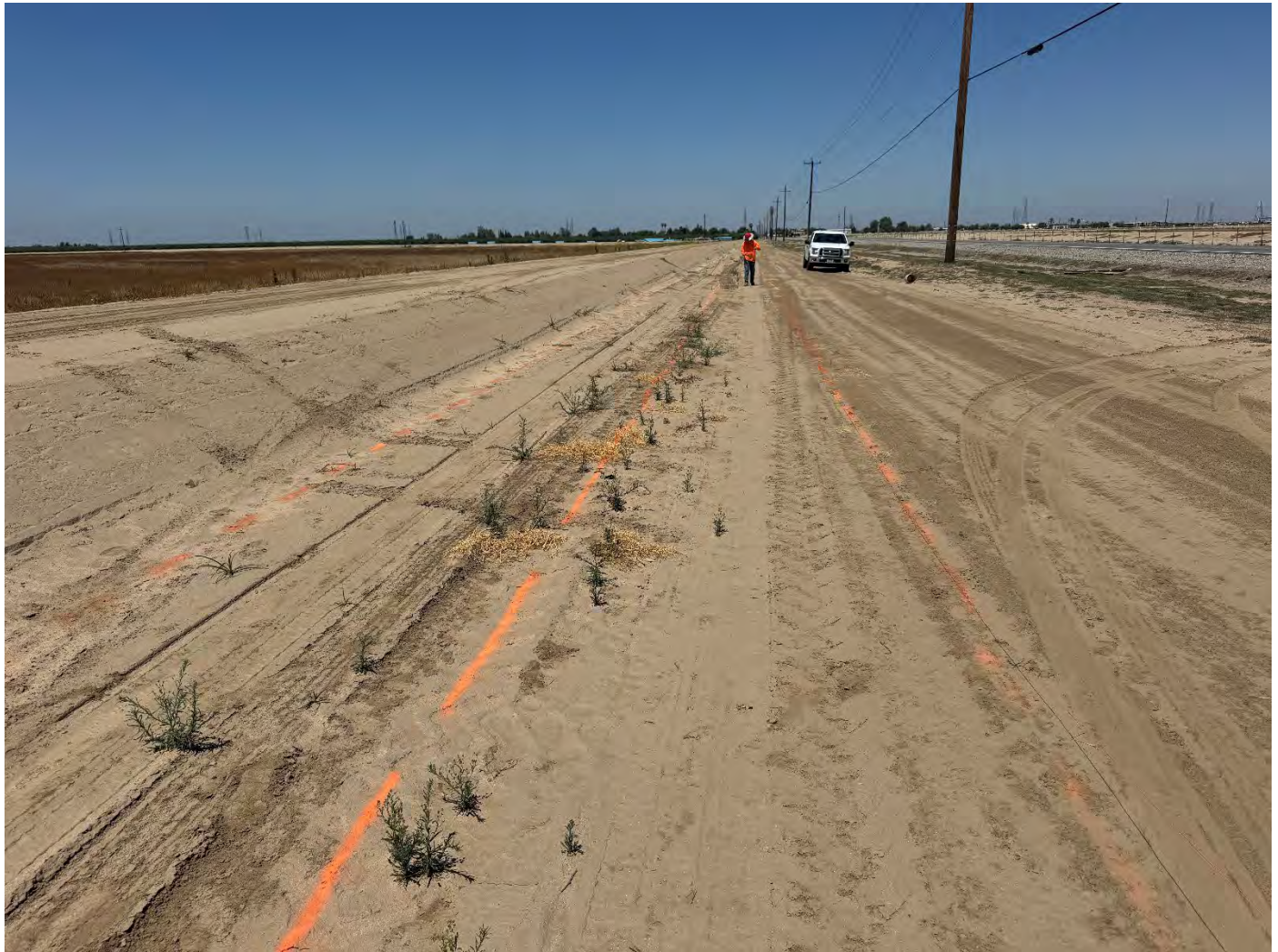
Excavator Track Boundary and Centerline of Pipeline Painted Along the Recovery Line Alignment
