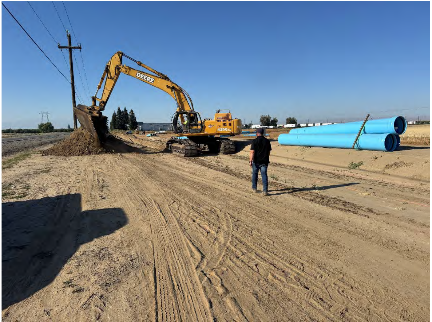
Excavating Trench Along Recovery Pipeline Alignment
