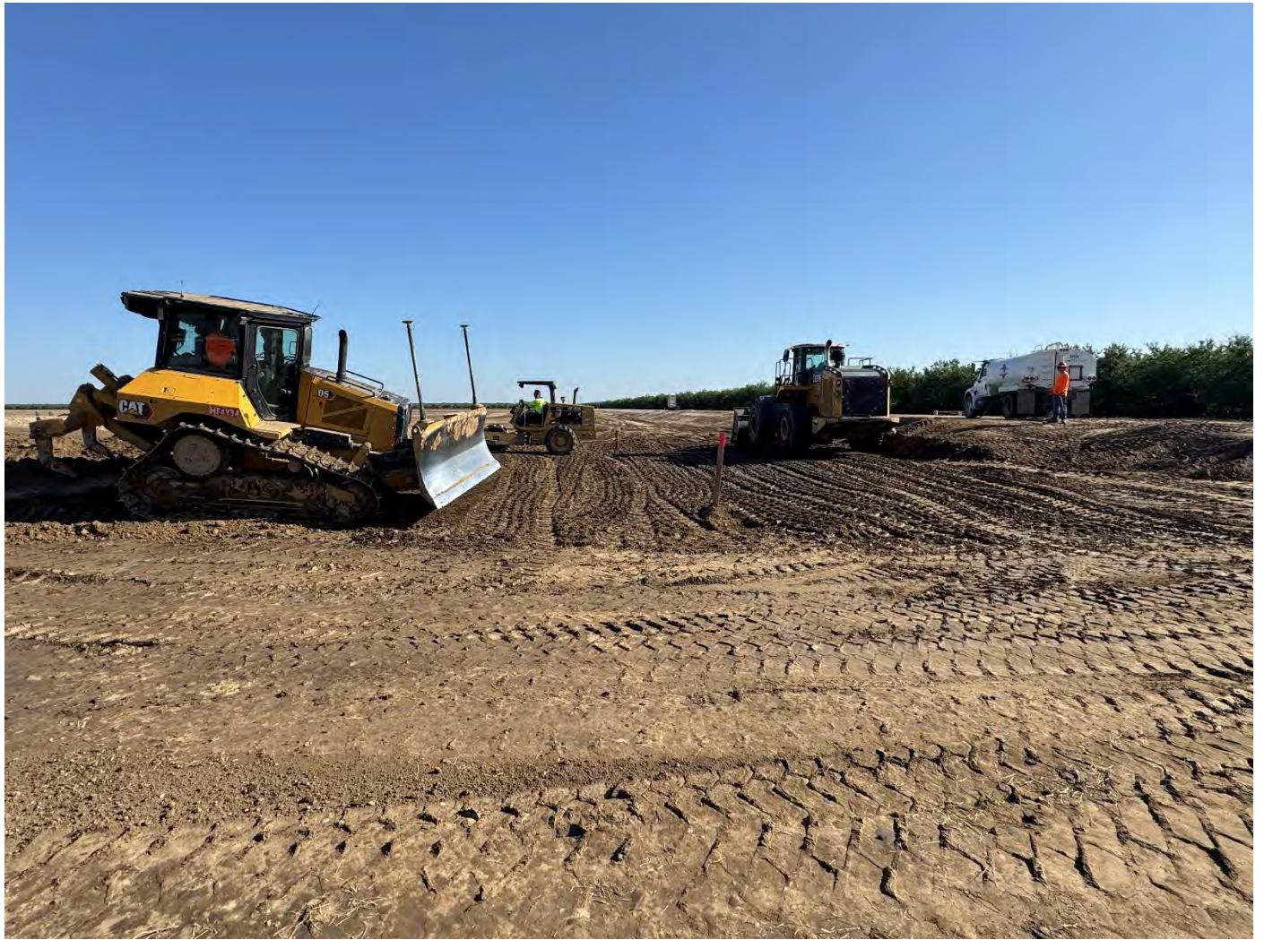
Earthwork at Embankment Near Cased Crossing
