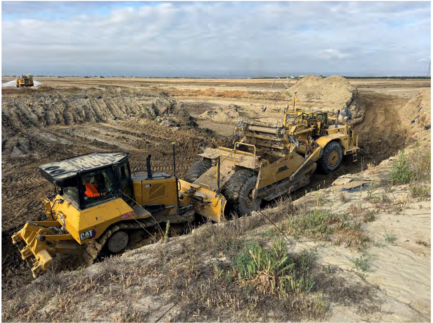
Excavating Existing Sump
