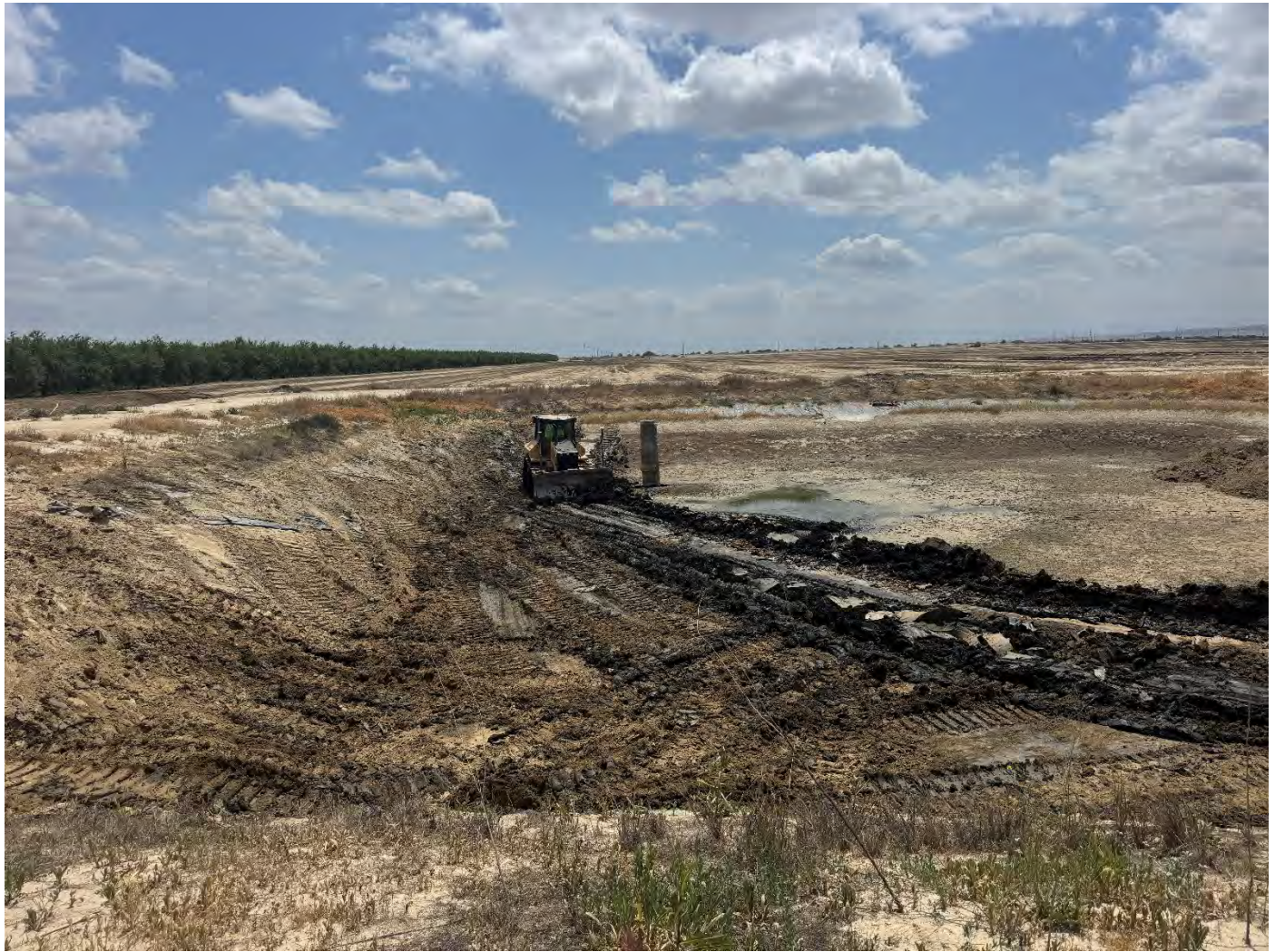
Progress Excavating the Sump and Removing Liner
