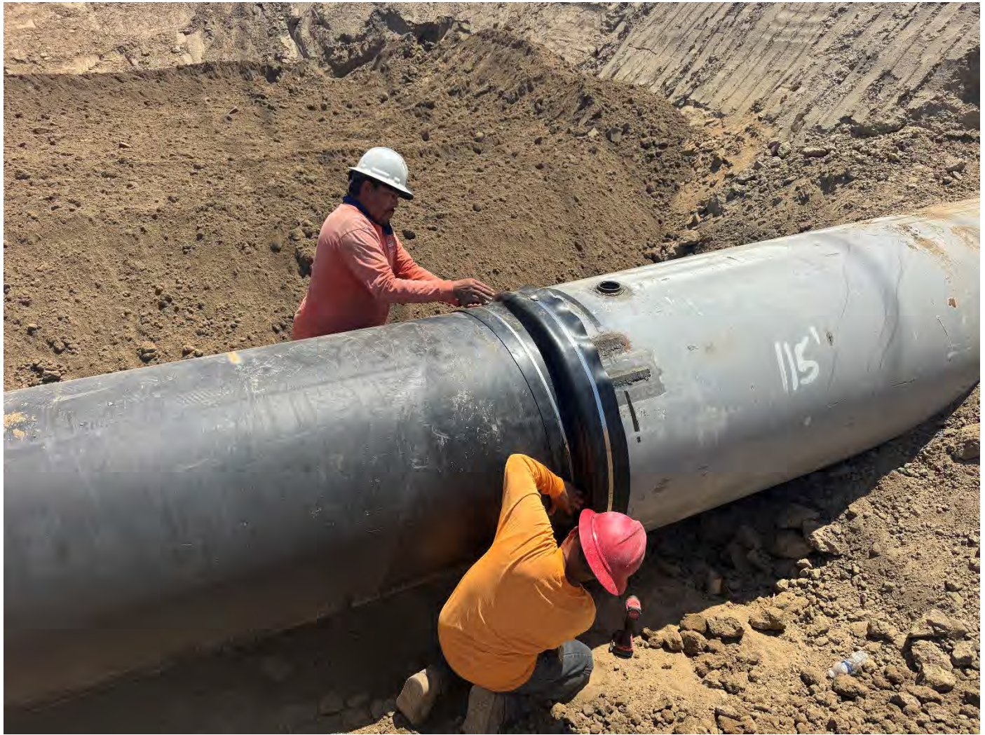
Installing End-Seal to North Side of Cased Crossing
