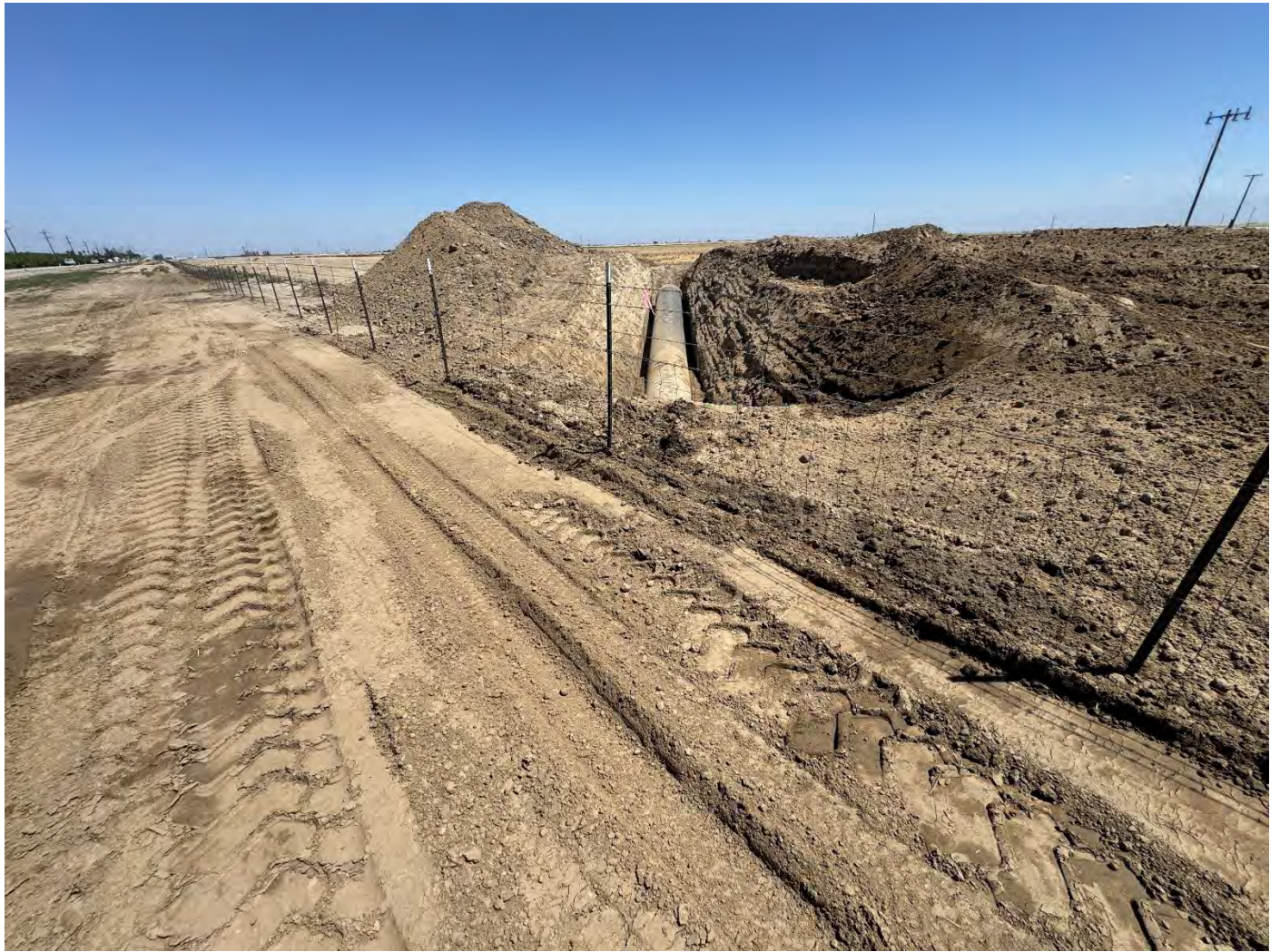
Pipe Trench Backfilled on South Side of Stockdale Highway
