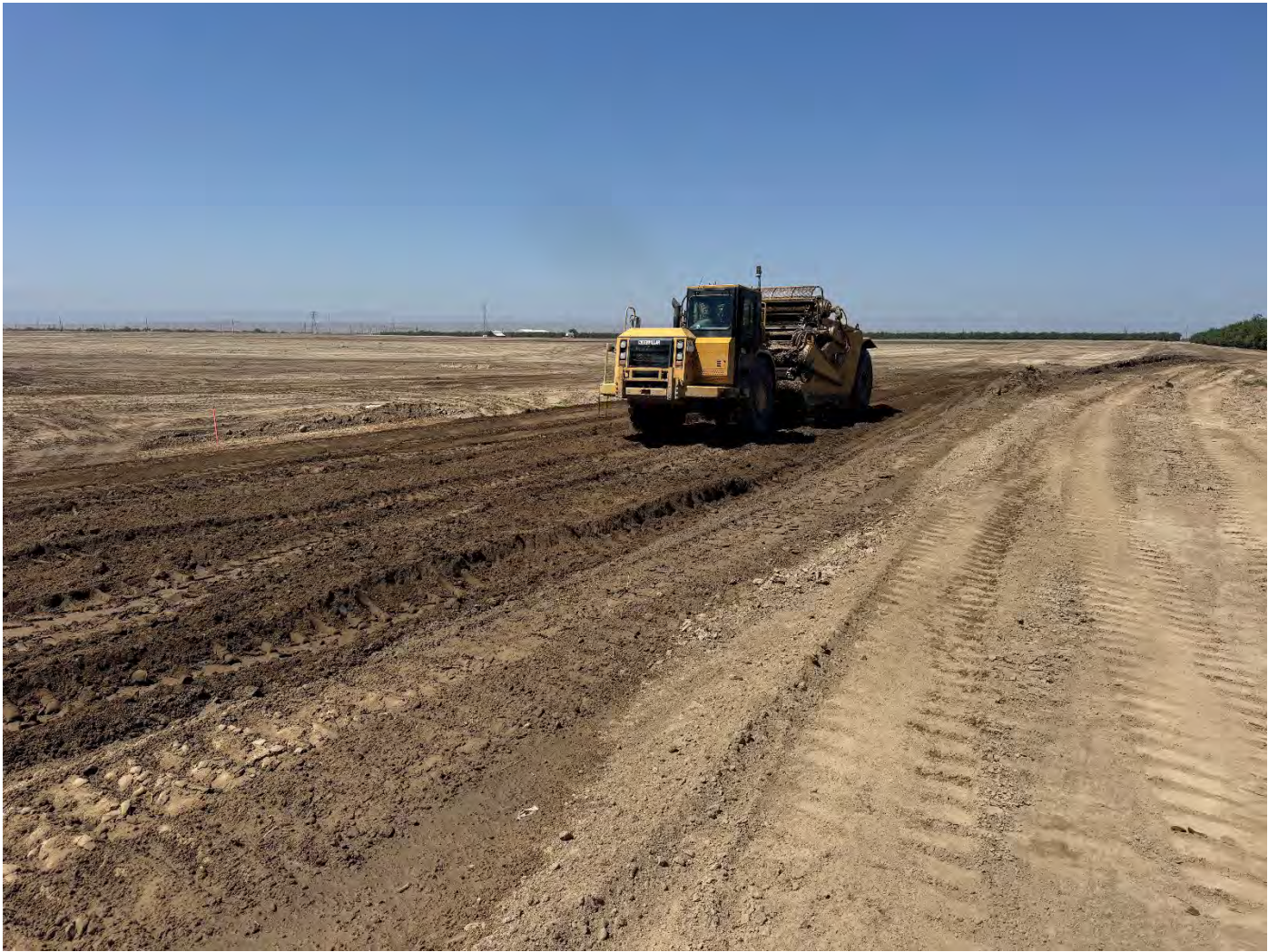
Backfilling Keyway at Northeast Corner of Property
