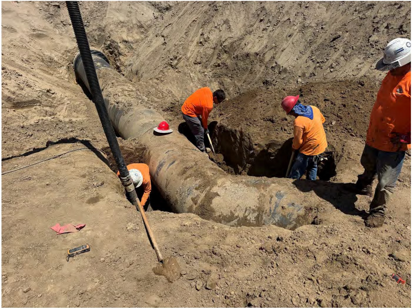
Concrete Thrust Block Bearing Area Excavated
