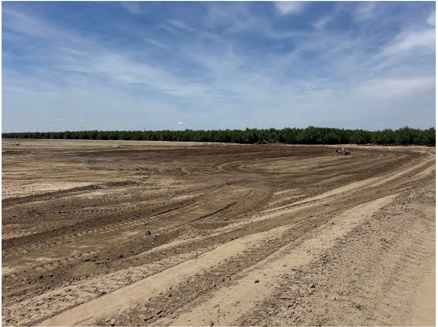
Existing Sump Removed; Excavating Keyway for Embankment
