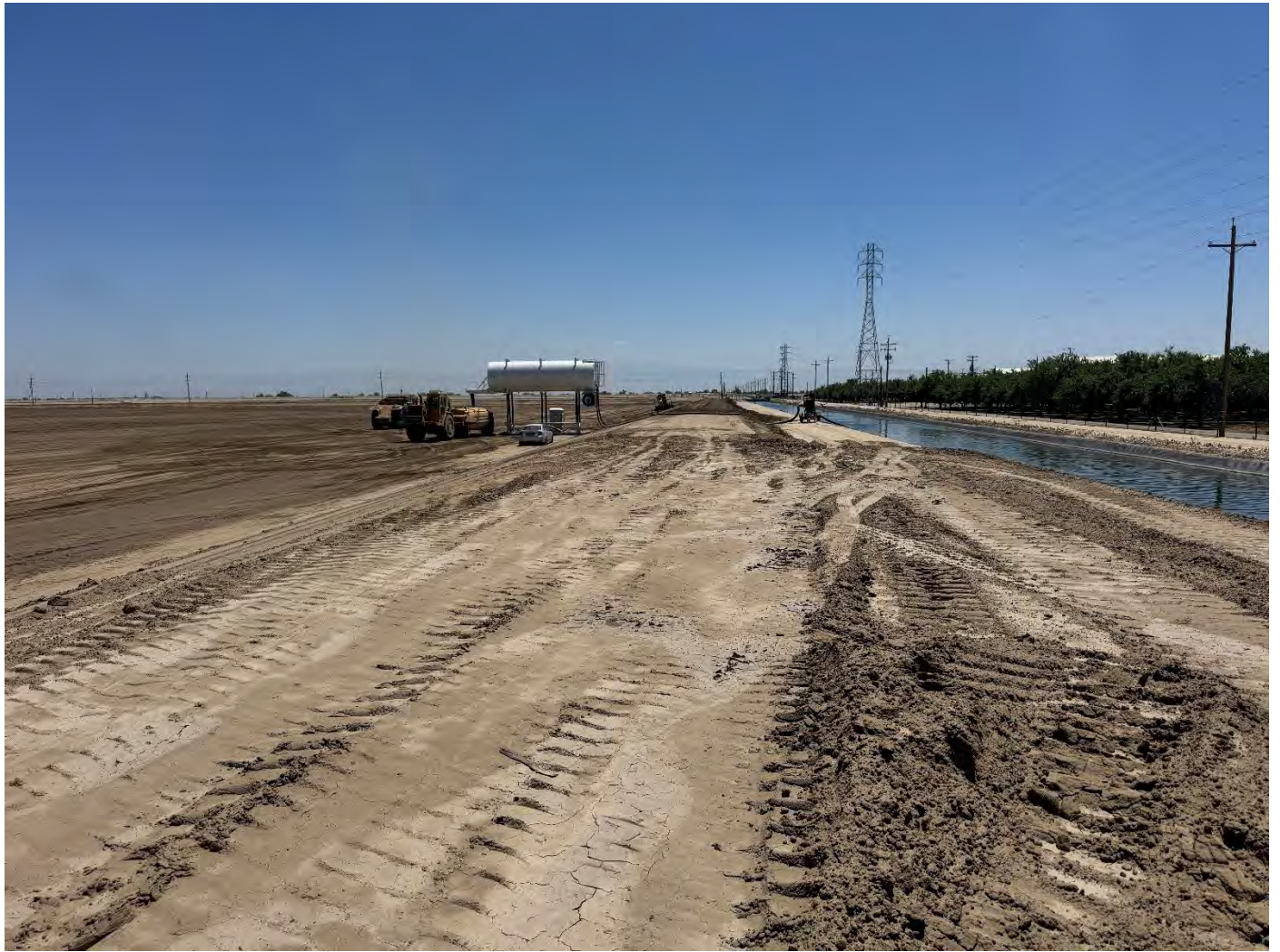
Fine Grading Embankments
