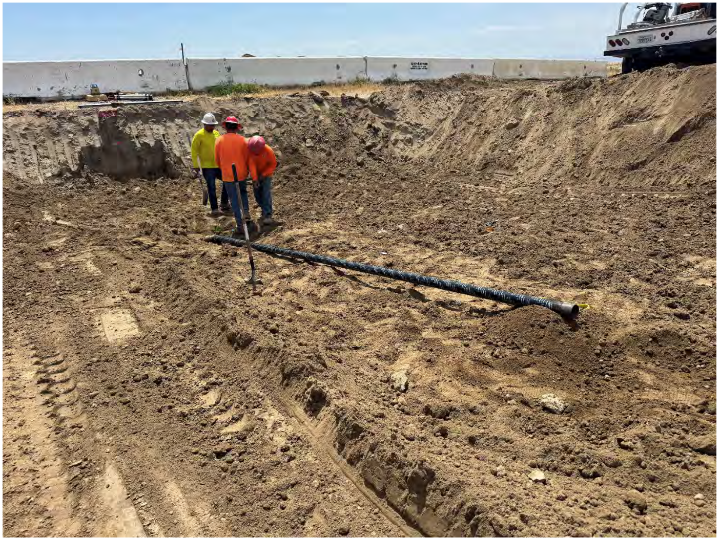
Backfill Above HDPE Pipe; Installing 3" Casing Vent Pipe
