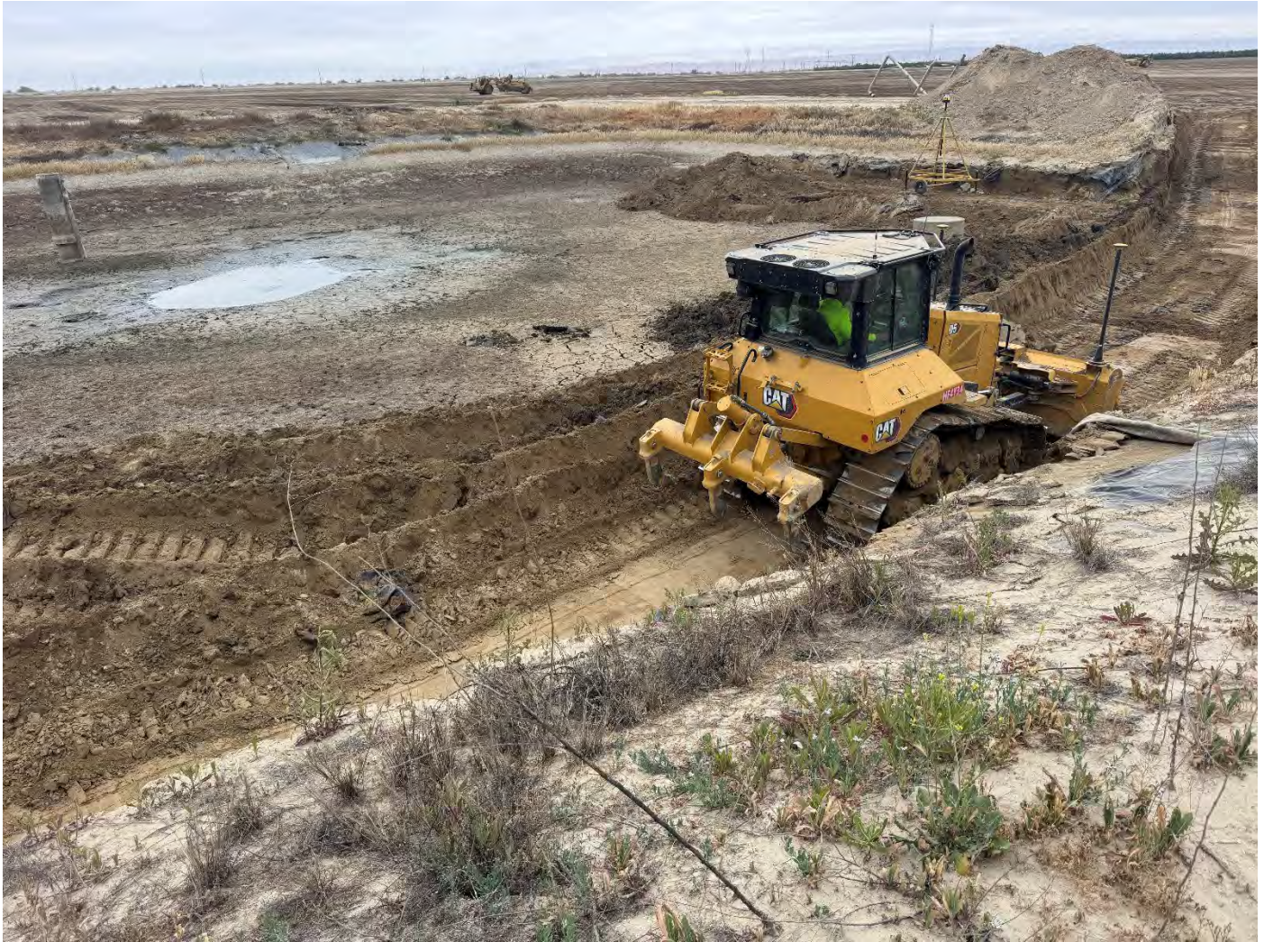
Excavating Existing Sump
