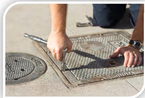
Grease Interceptor is Opened for Inspection
