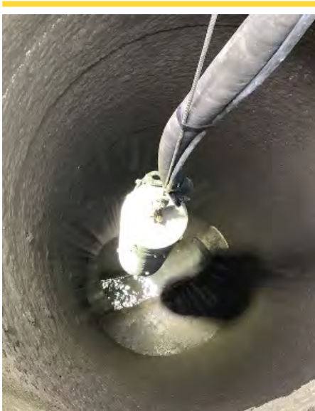
Spin casting, a type of SIPP, can be used for remotely rehabilitating vertical sections of varying diameter pipe.
