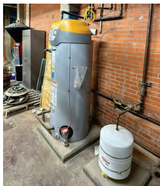
Natural gas fueled water heater and pump.
