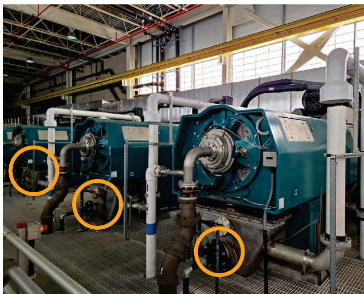
Existing Tortuous Path for TS Flow
