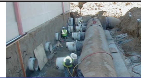
EARL SCHMIDT INTAKE PUMP STATION MODIFICATIONS SANTA CLARITA VALLEY WATER DISTRICT
