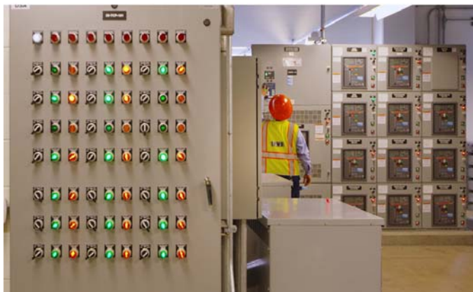
Employee working in Electrical Room
