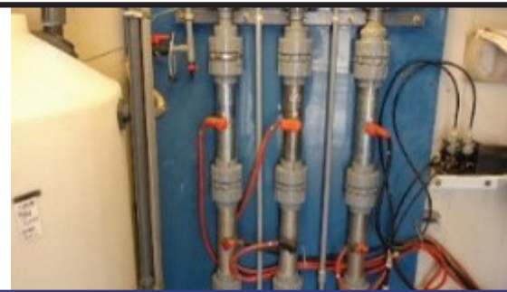
2016-2017 RESERVOIR MANAGEMENT SYSTEMS REPLACEMENT PROJECTS MOULTON NIGUEL WATER DISTRICT
