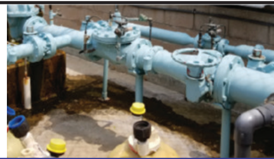
ESTADO RESERVOIR MANAGEMENT INSTALLATION SYSTEM SANTA MARGARITA WATER DISTRICT
