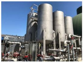
Test and/or replace pressure vessel safety valves (PSV) as needed during annual shutdown.
