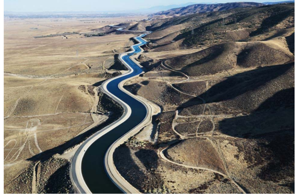
California Aqueduct, SWP
