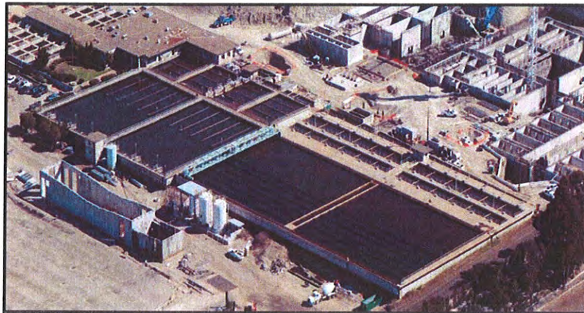
Figure 5-1: Typical Flocculation-Sedimentation Basins
