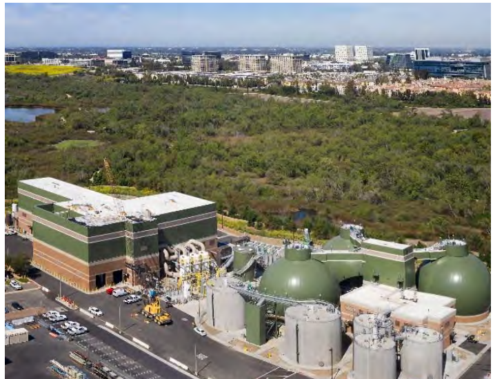
Biosolids and Energy Recovery Facilities
