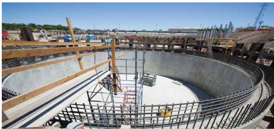
Biosolids and Energy Recovery Facilities Project
