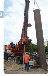
A crane is used to lower the conductor casing into a newly-drilled borehole. This casing will stabilized the borehole.
