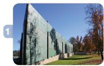
The sound curtains erected around a drilling site help buffer drilling noises and mask the drilling in progress for nearby residents and businesses.
