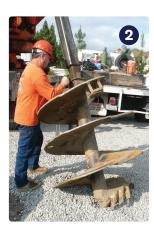
In preparation for borehole drilling, the bucket auger drill is attached to a drill rig.
