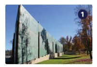
The sound curtains erected around a drilling site help buffer drilling noises and mask the drilling in progress for nearby residents and businesses.
