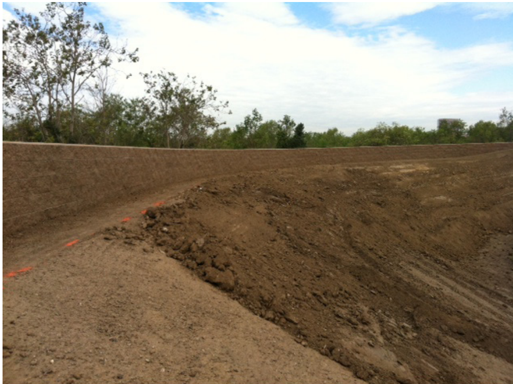
Figure 3.1-3: View of Flood Wall and Berm
