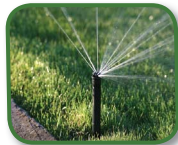
Rotating nozzles direct spray streams more accurately away from pavement.
