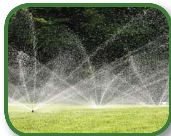
Install rotating nozzles on all spray heads operated by the same valve.
