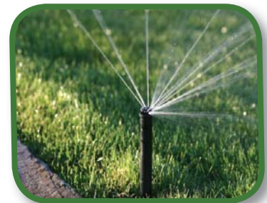
Spray streams are more accurately directed away from pavement.
