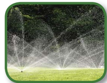
Install rotating nozzles on all spray heads operated by the same valve.
